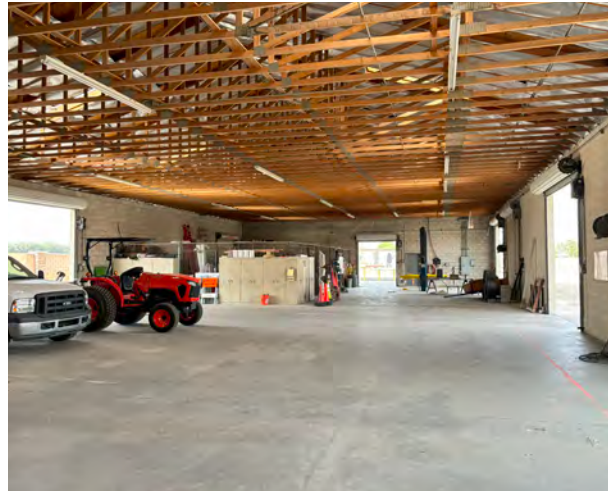
Figure 15: Warehouse-Style Operations Building with Offices in the Back
